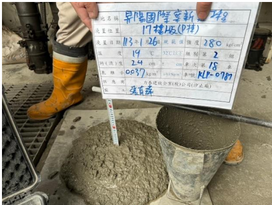
混凝土坍度試驗
