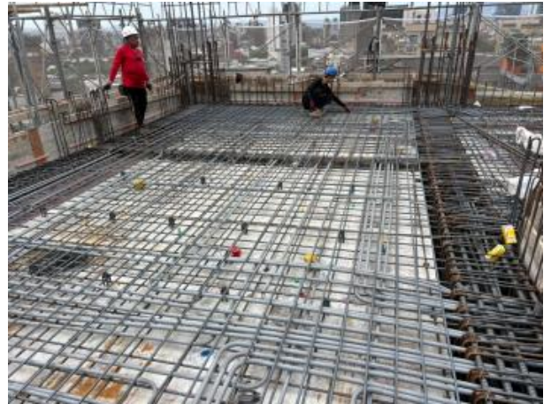
12FL梁板筋綁紮
