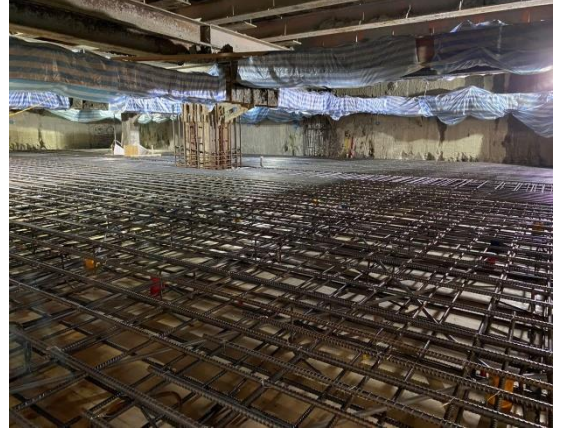
B1FL鋼筋綁紮
